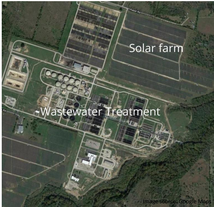
Solar farm located at wastewater plant
